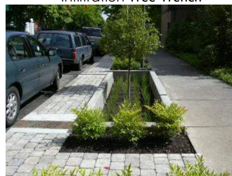
Infiltration Tree Trench
