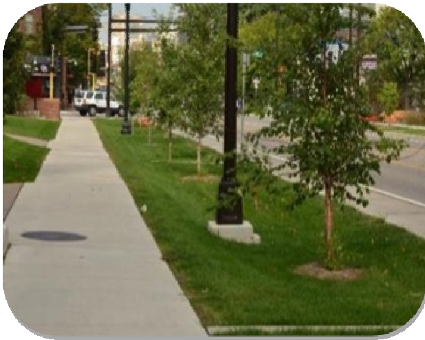
Exhibit 4.2.6A/B: Example Grassed Swale & Biofiltration
