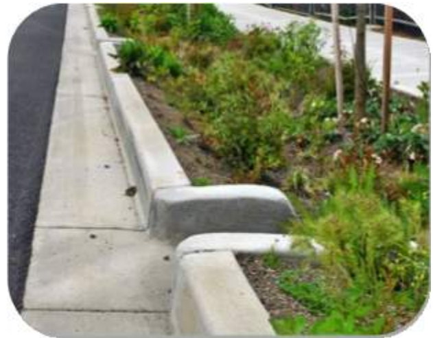
Exhibit 4.2.9D: Bioswale Curb Cut
