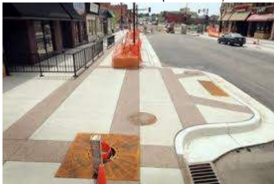
Green Infrastructure Infiltration Trench
